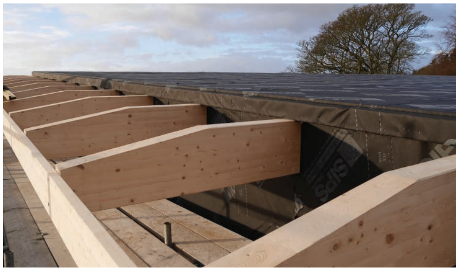
The SIPs roof design incorporates a 5° monopitch metal roof folding down the back and around the house.
